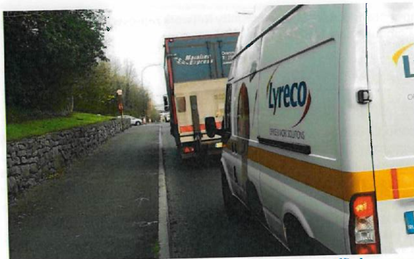
Figure 1: Photograph showing the impact that using a 3.2m traffic lane on an arterial road has on road space for people on bicycles. Location: Tuam Road, Galway.
