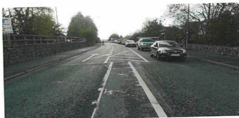
Figure 2 Photograph showing the impact that using a 3.2m traffic lane on an arterial road has on road space for people on bicycles. Location: Tuam Road, Galway.
